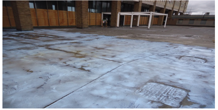
Podium deck primed with Flexcrete EF Primer in readiness for application of Cemprotect Elastic
