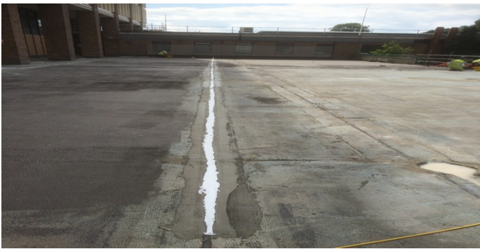
Cemprotect 2000S bandage system applied over in-situ movement joints.
