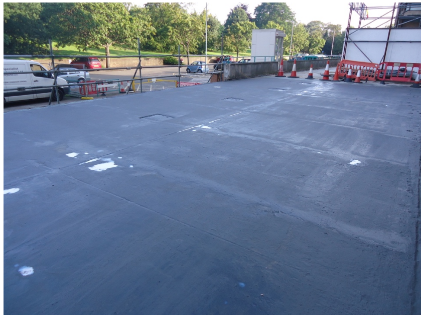
A section of the podium deck following the application of the Flexcrete Cemprotect Elastic waterproofing system
