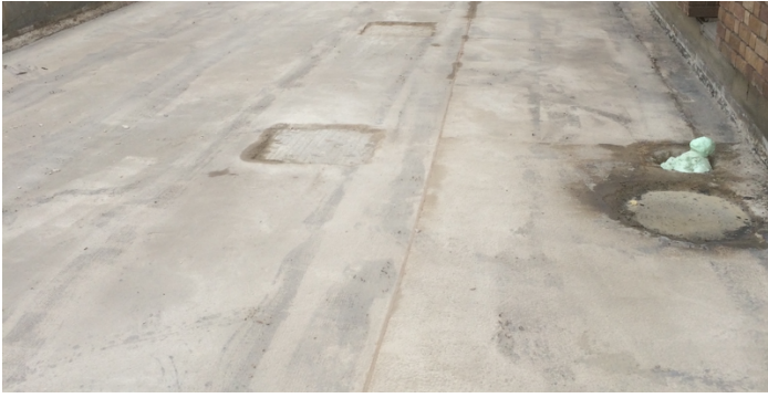
An area of podium deck scabbled in preparation for waterproofing application
