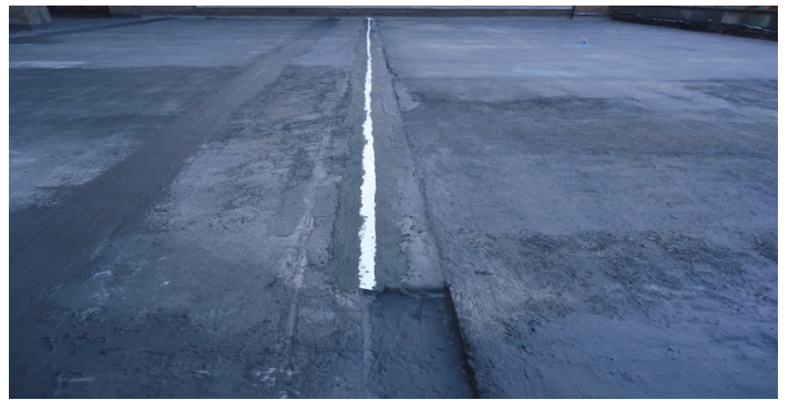
Cemprotect 2000S both in the finished over-coated state (left), and installed yet exposed in preparation for over-coating (right)
